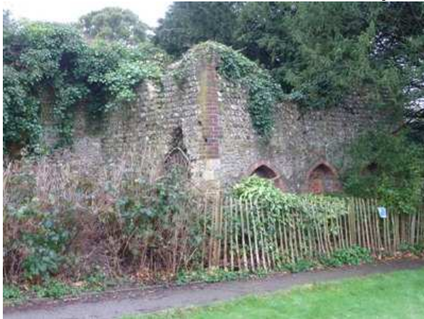
Preston Well House in state of disrepair
